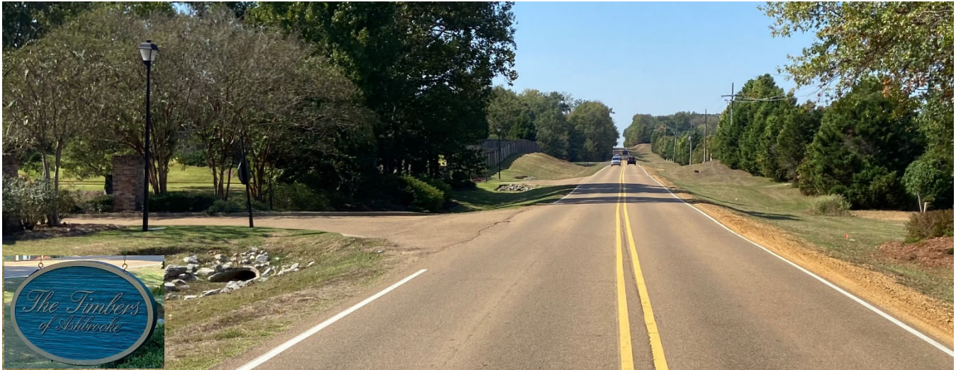
Above: Looking west along Stribling Road at Timber Drive.
